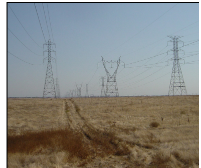
The WAPA corridor's power lines and related towers crossing the SVSP.
